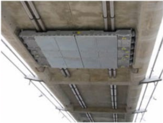
Mass damper on the underside of a bridge
